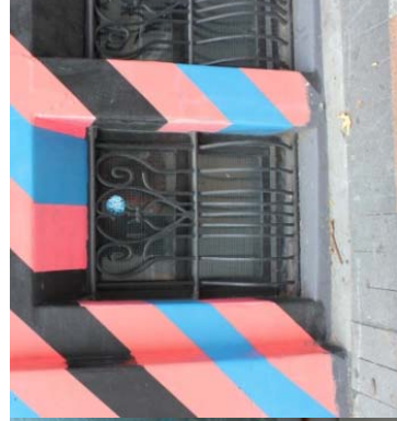
Wrought iron window screen
